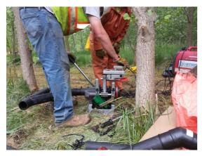
Conveyance piping was run from PW-2 to ECB-2. A clean-out fitting was installed at the well head and at the ECB to allow for line jetting from either direction. At the ECB, piping installed above 36 inches below grade up to the ECB entrance were heat-traced and insulated to prevent freezing.
